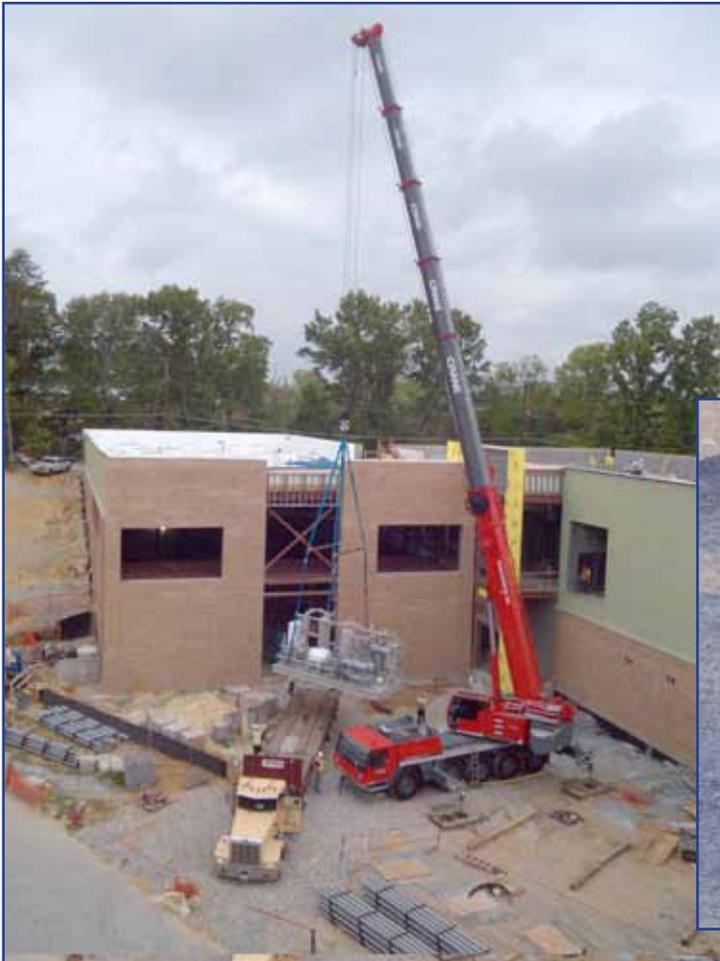
(Left) On May 7, Pierce and Crane Rental rigged 3 gas compressors, 2 blowdown tanks, and 2 de-aerators into the FDA CUP Expansion. Shown to the left is one of the three gas compressors being craned into the second floor service opening.
